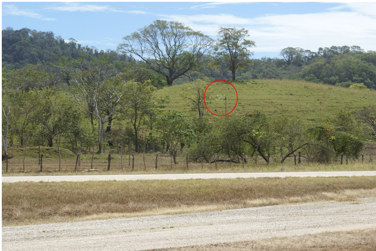
Figure 8 – Windsock structure at departure end of runway 03 at MRIA with missing windsock on the day following the accident.
