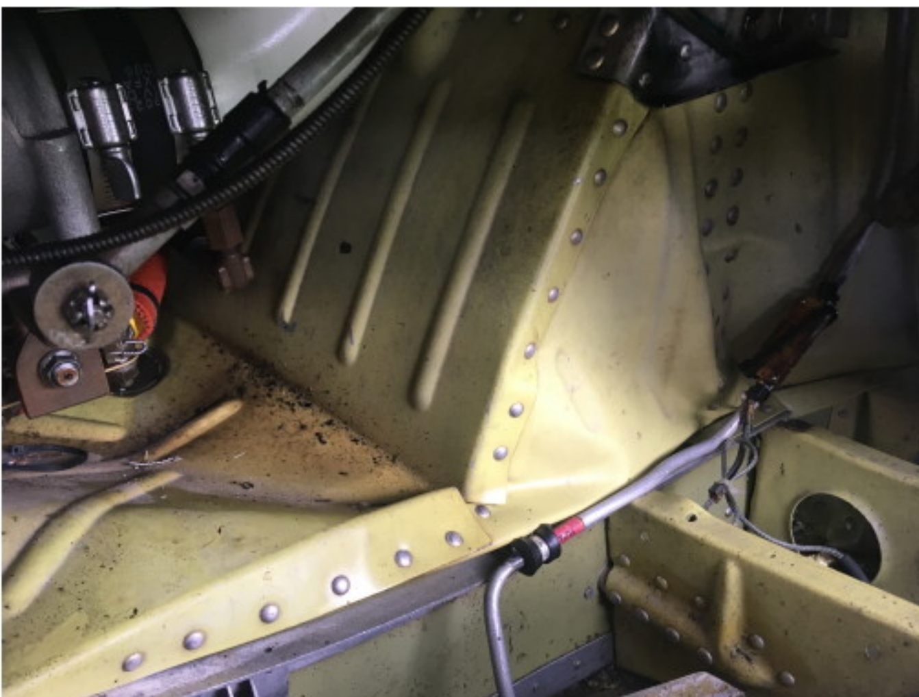
Keel and Support structure
