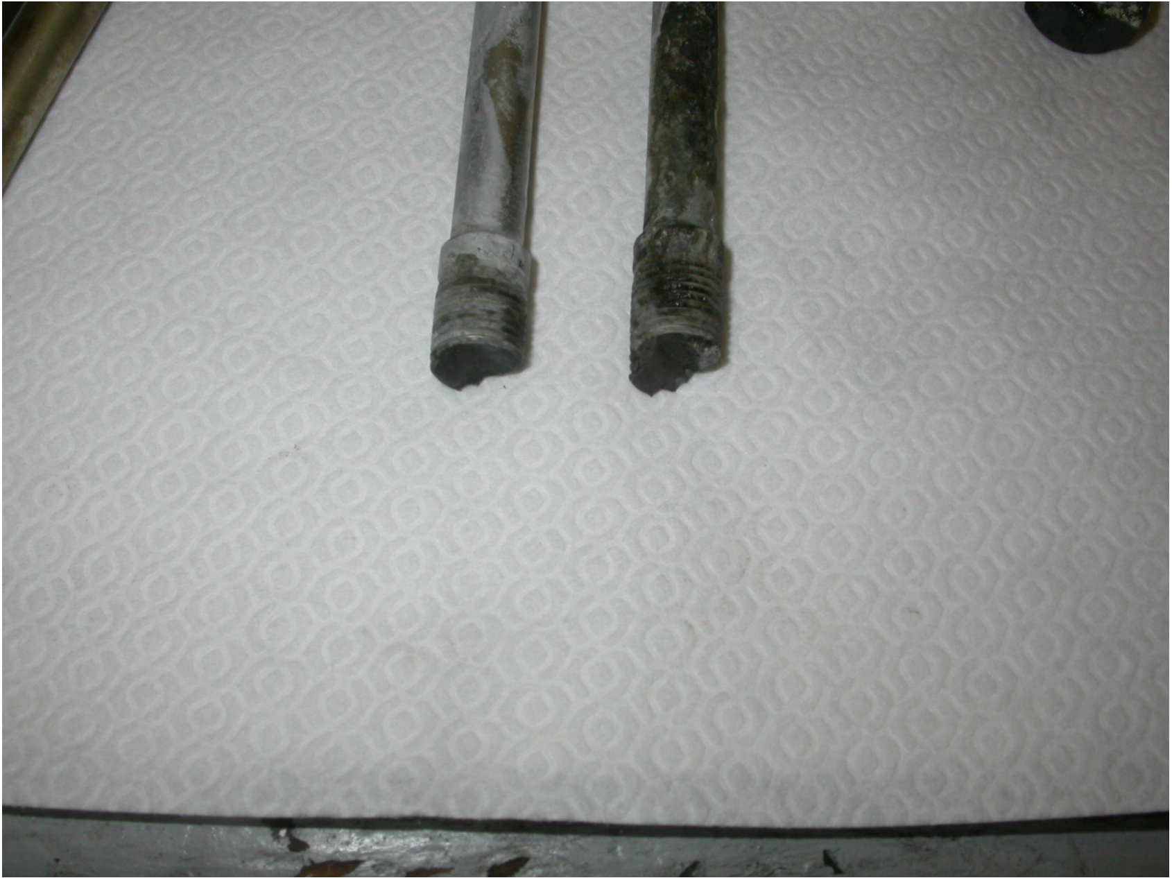
Photo 31 – View of 2 fractured through bolts
