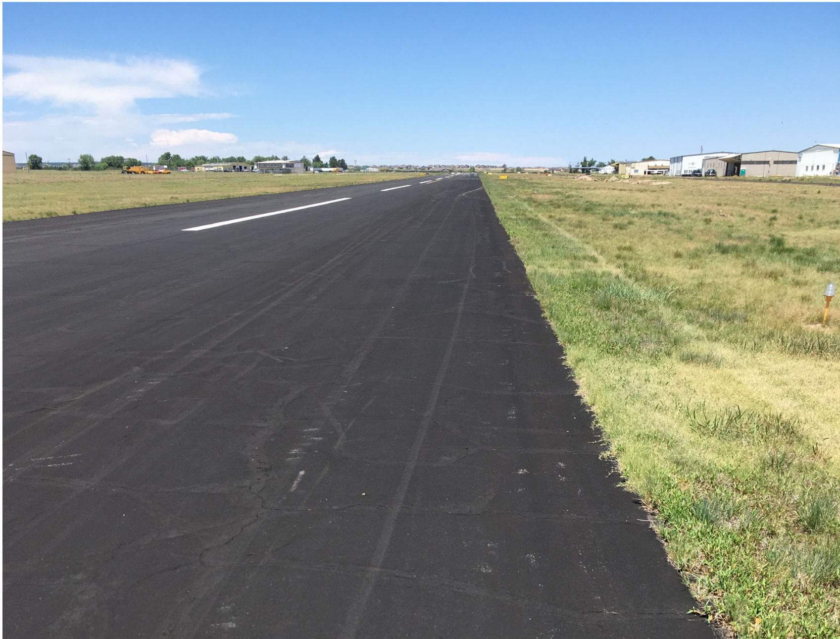
Photo 3 – Runway Witness Marks
