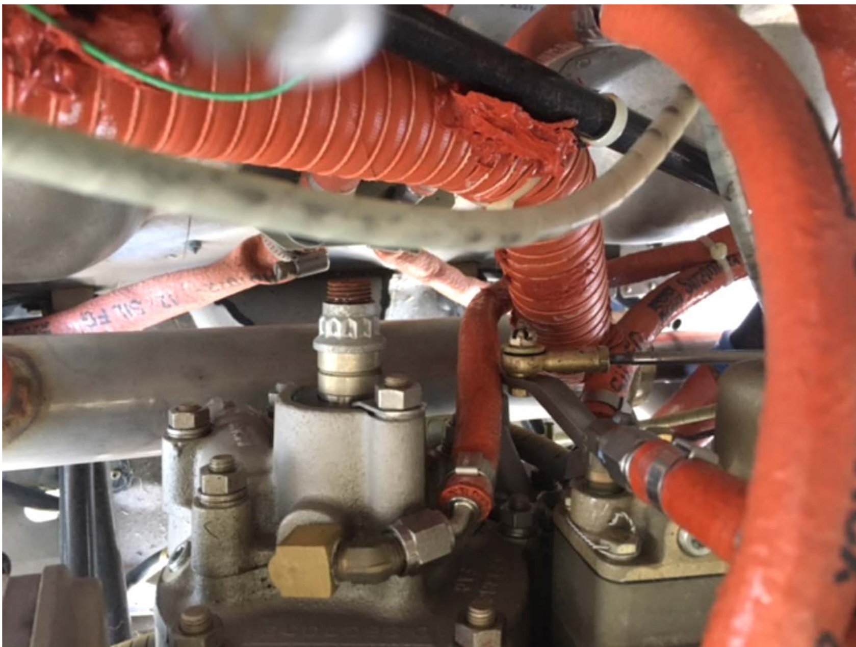
Photo 1 – View of hose routing on N9306 (accident airplane)
