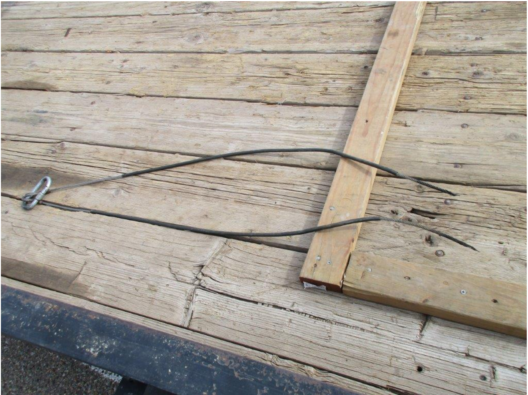
Photo 4 – Second Suspension Cables Damage
