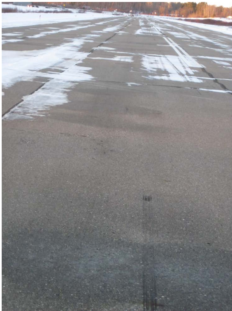
Photo 9 - Supplied close-up photo of runway witness marks with the accident airplane in the background.
