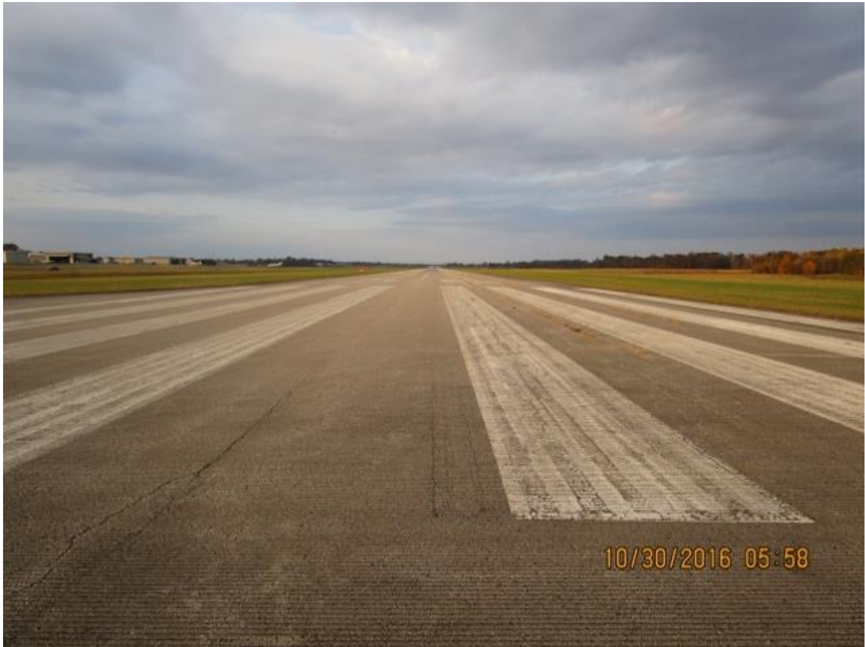
Photo 2 – View of the end of runway 18
