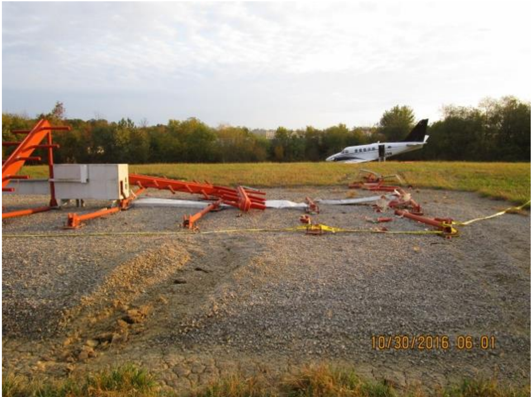
Photo 4 – View of the damaged ILS structure damage
