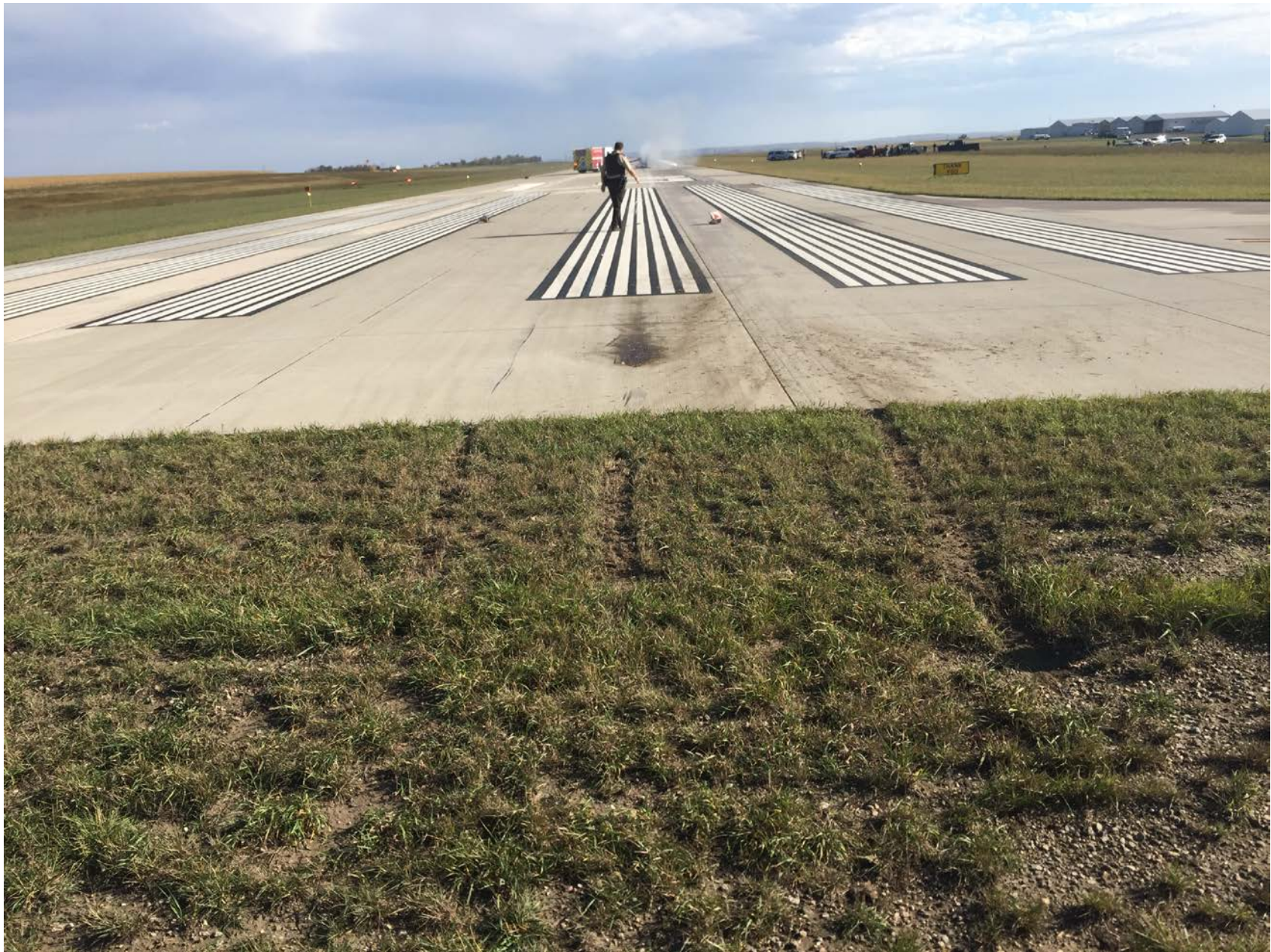
Photo 4 – Accident Site View Down the Runway
