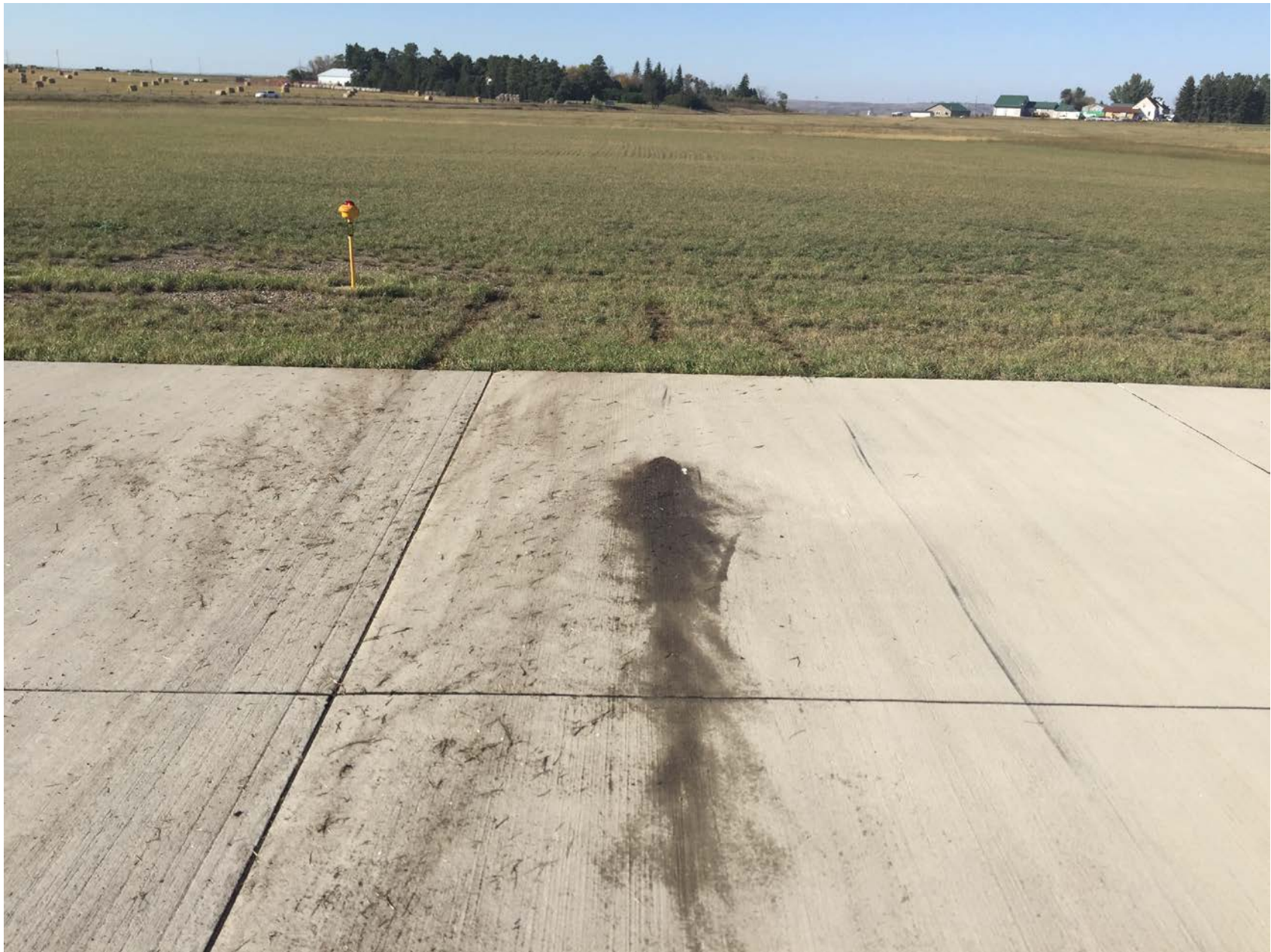
Photo 2 – Accident Site Landing Gear Impressions Short of Runway
