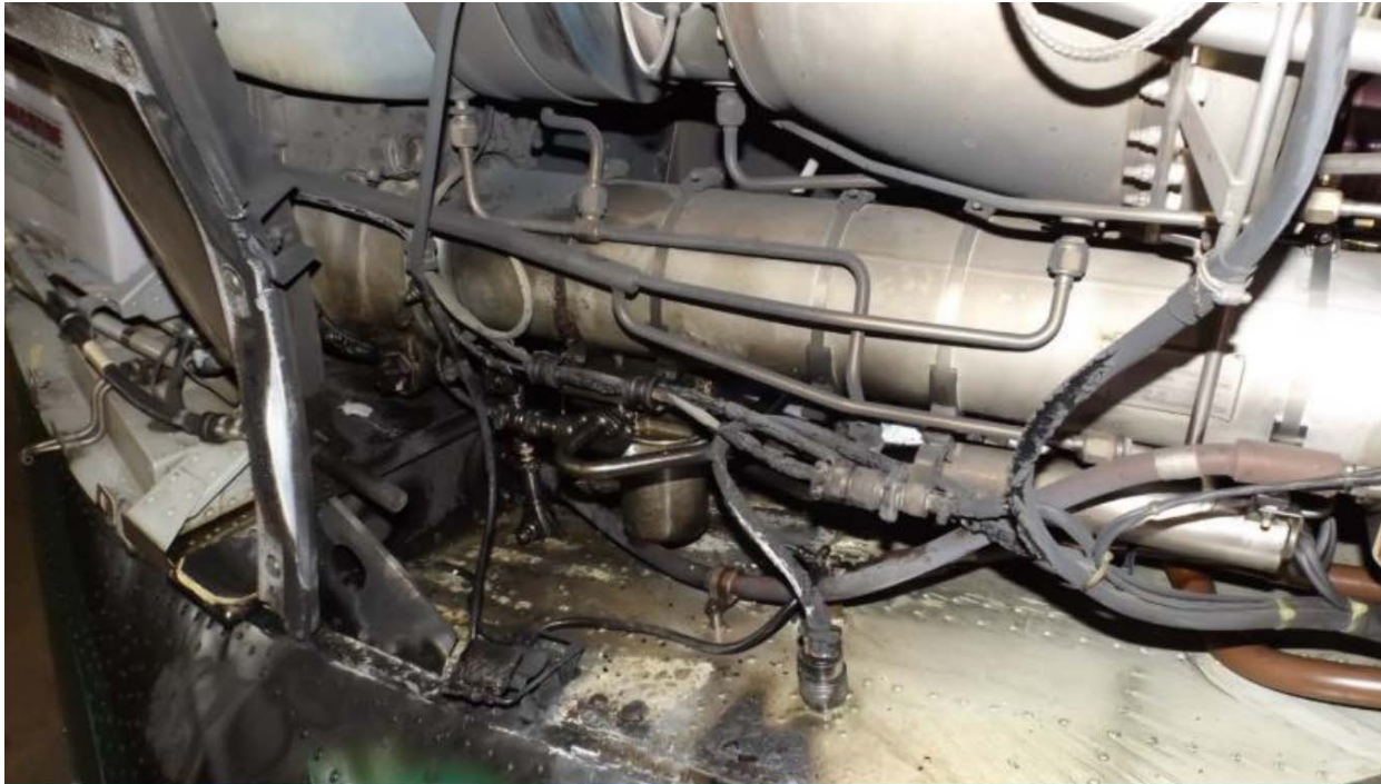
Figure 3 – No. 2 engine deck fire damage
