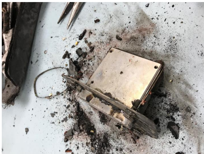
Figure 3. Photo of damaged RDM.
