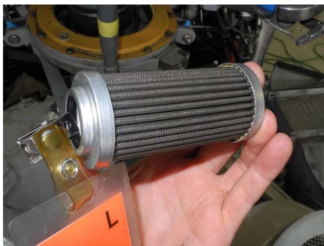
Figure 8. No. 1 engine fuel filter.
