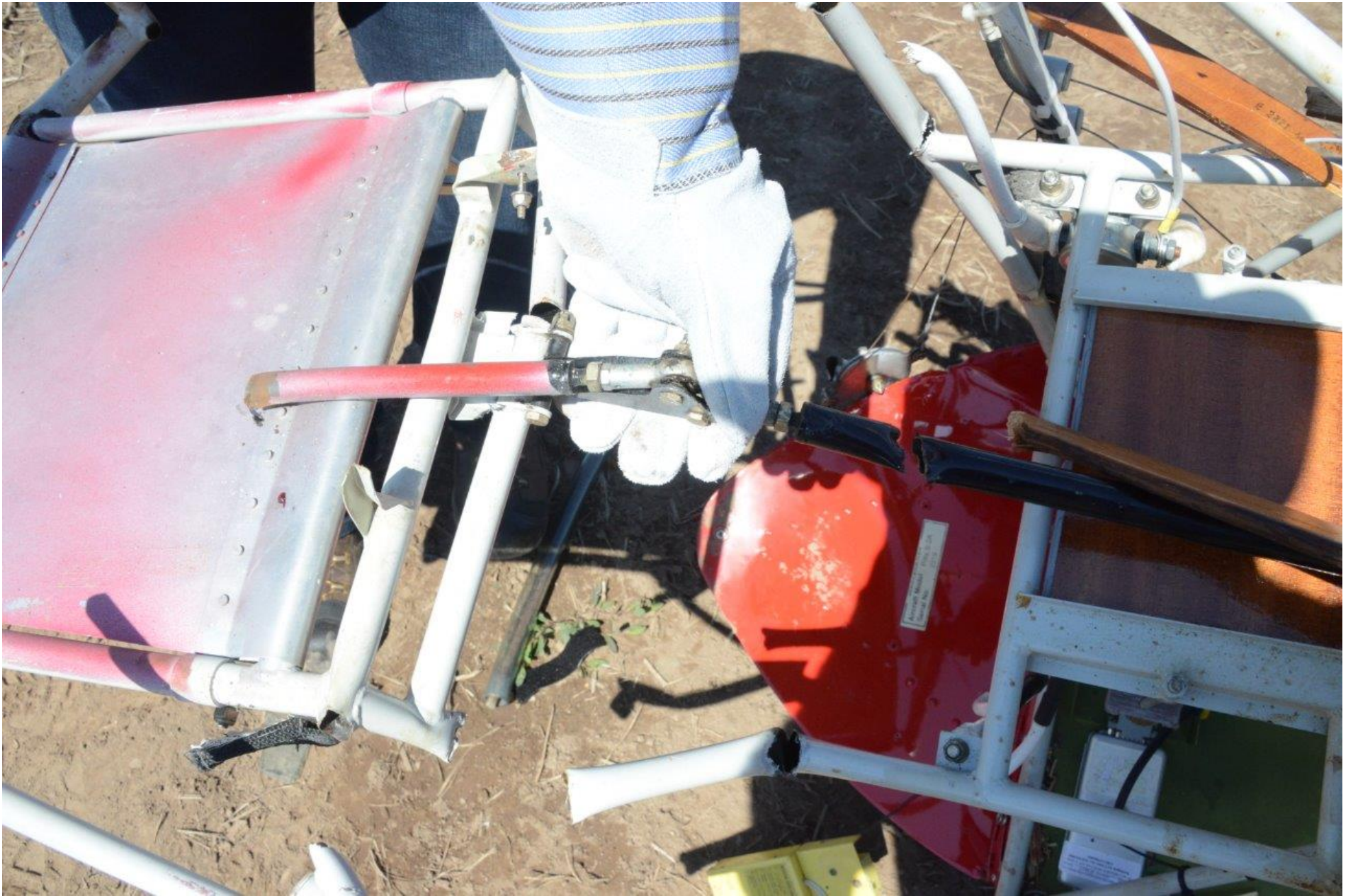
Photo 6 - View of separations in the push pull tubes.
