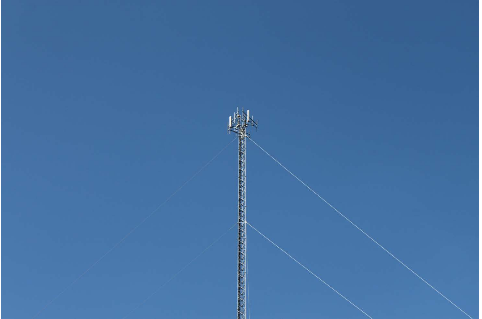
Photo 2 – Top View of Communications Tower
