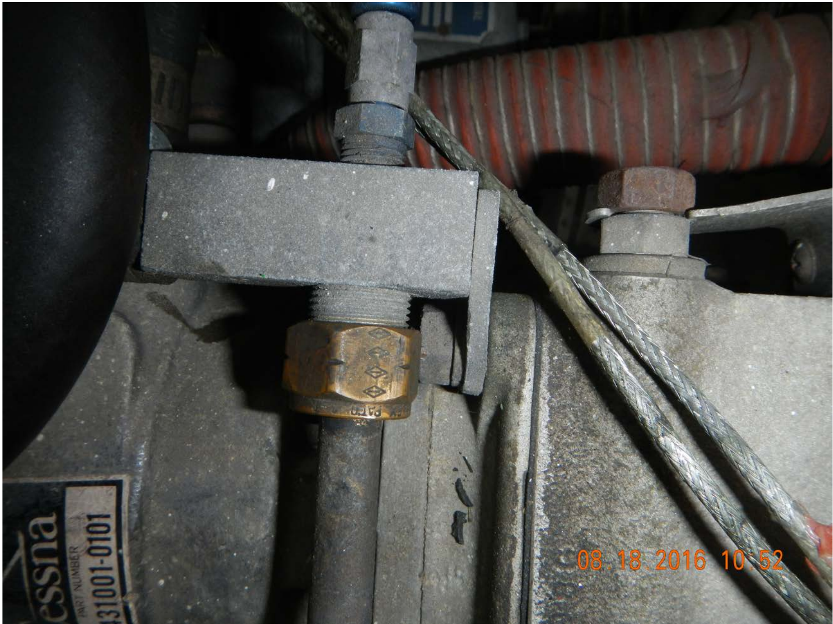
Photo 6 - Closeup of Loose B-Nut Fitting
