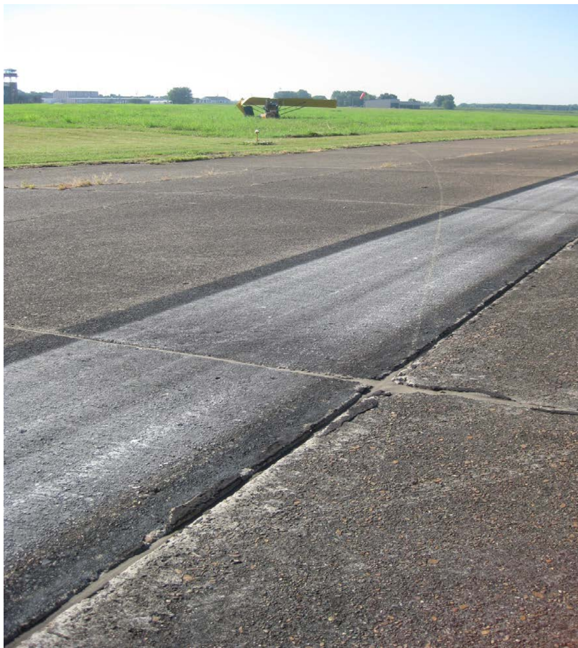
Photo 1 – Accident Site and Runway
