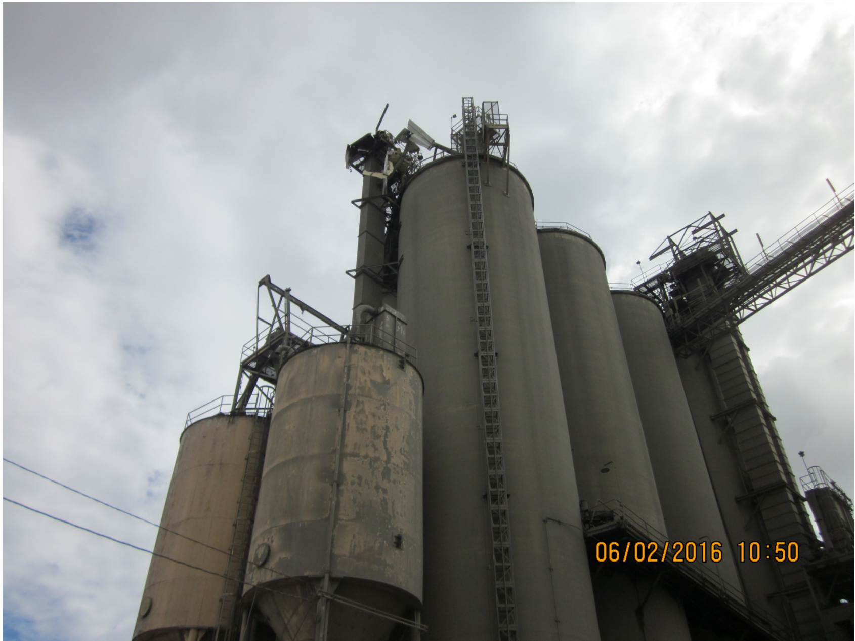
Photo 1 – The wreckage of N5679G embedded in the top of a 138-foot tall concrete silo.
