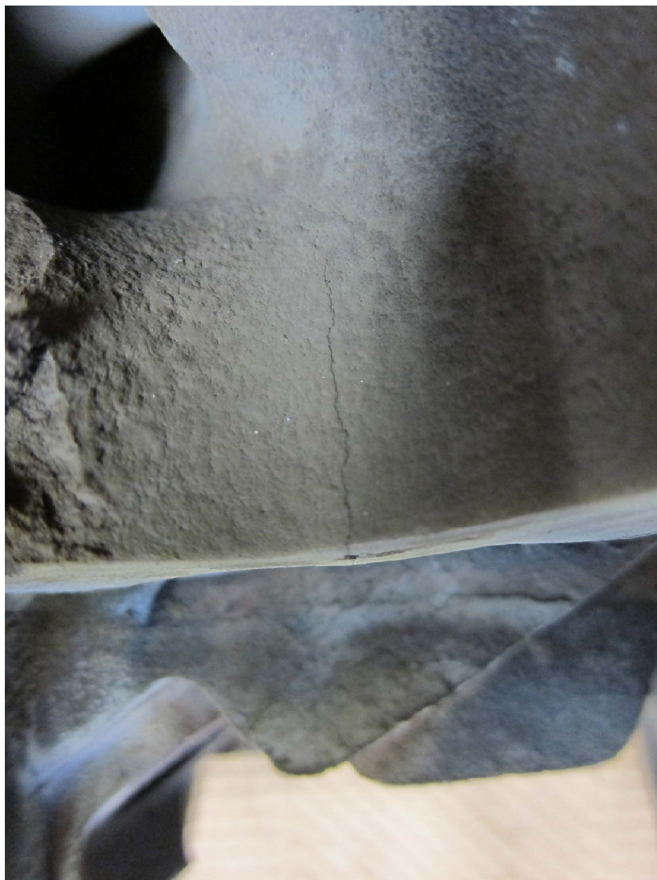
Photo 3 – View of Number 4 Cylinder Crack
