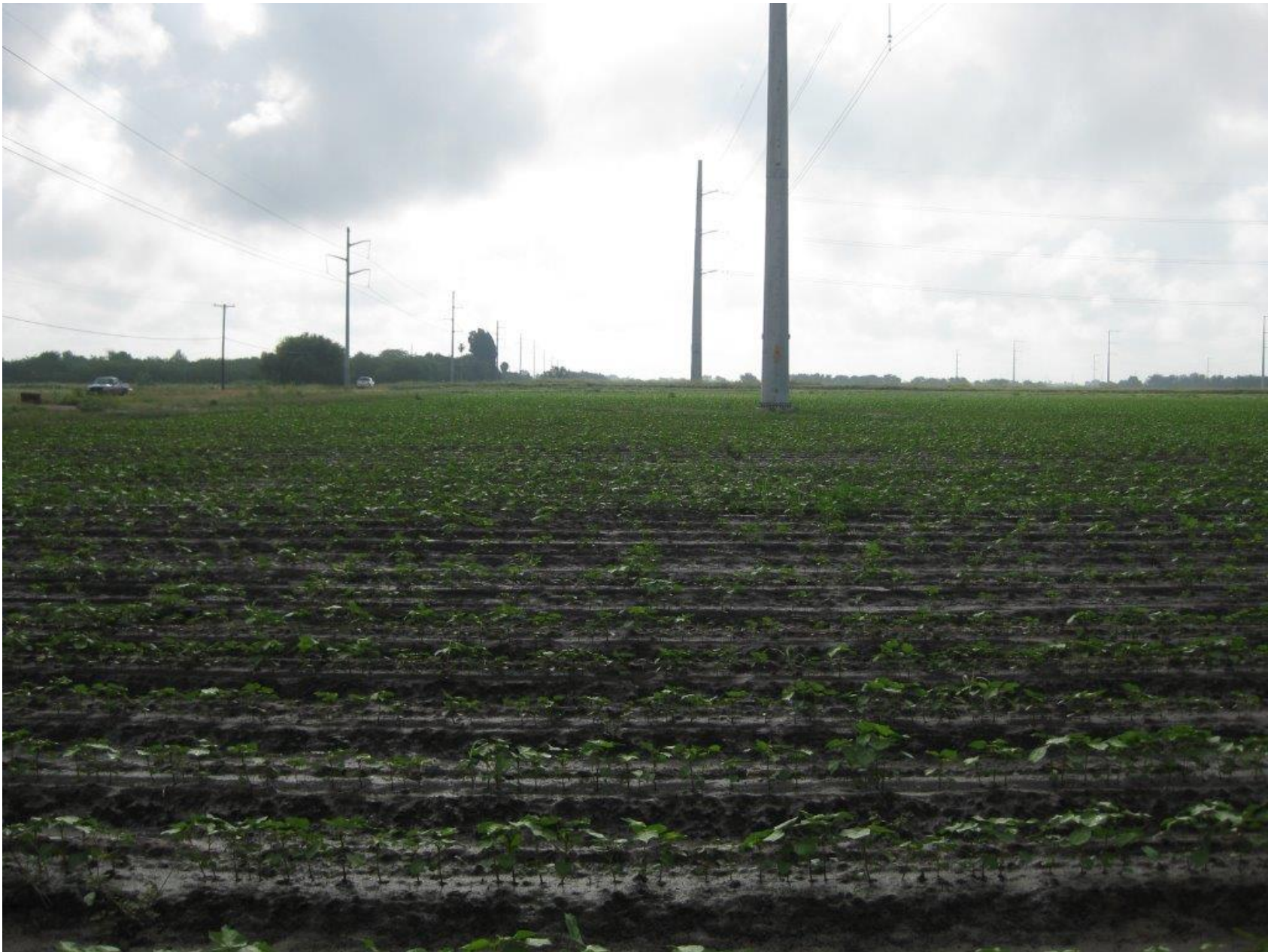
Photo 1 – Power lines that were struck by N64702.
