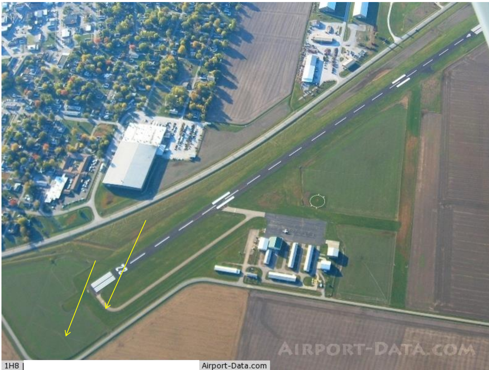
Photo 14 – Casey Municipal Airport, Parallel Taxiway and Perimeter Road
