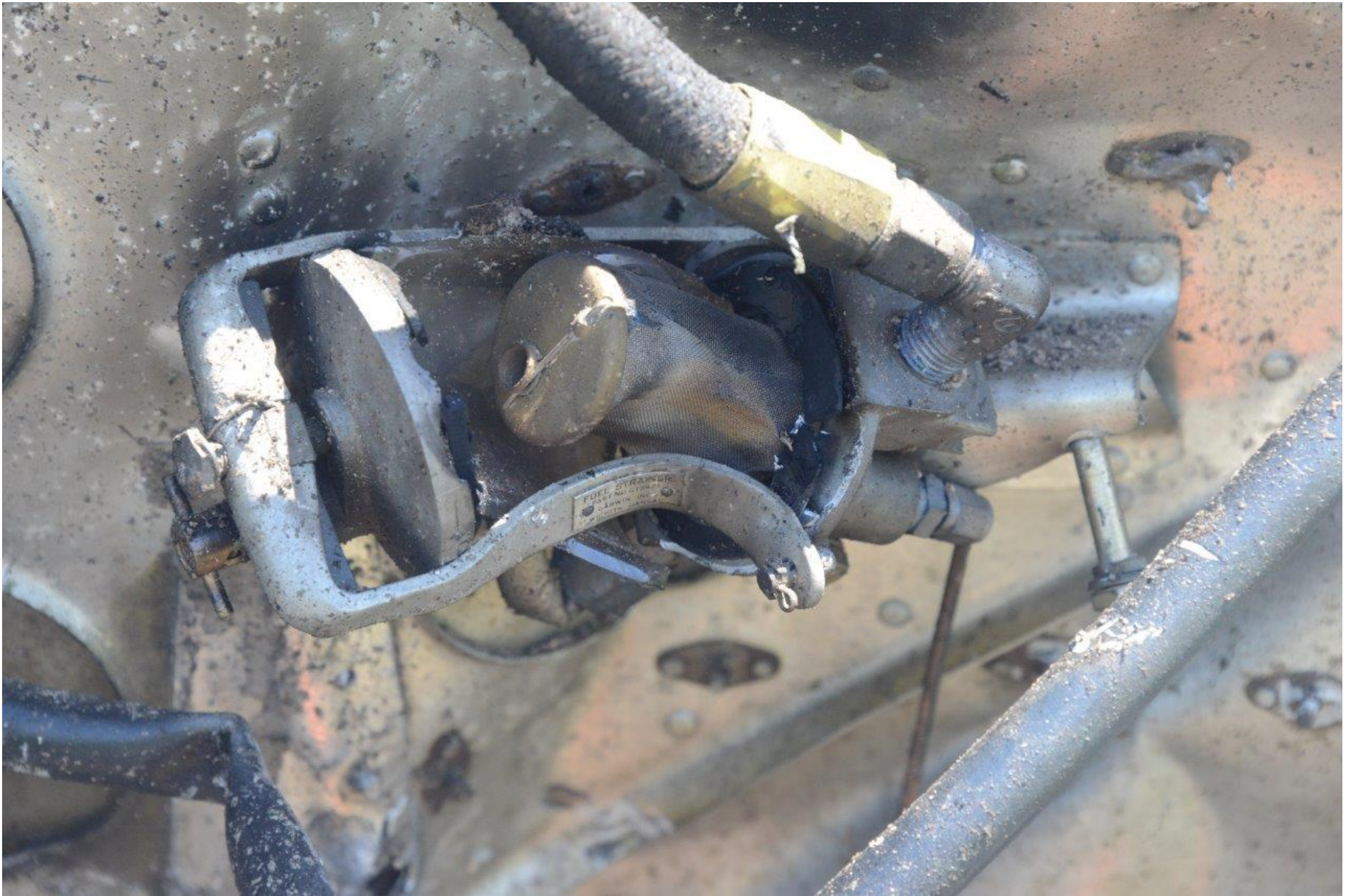
Photo 6 – View of the fuel strainer.
