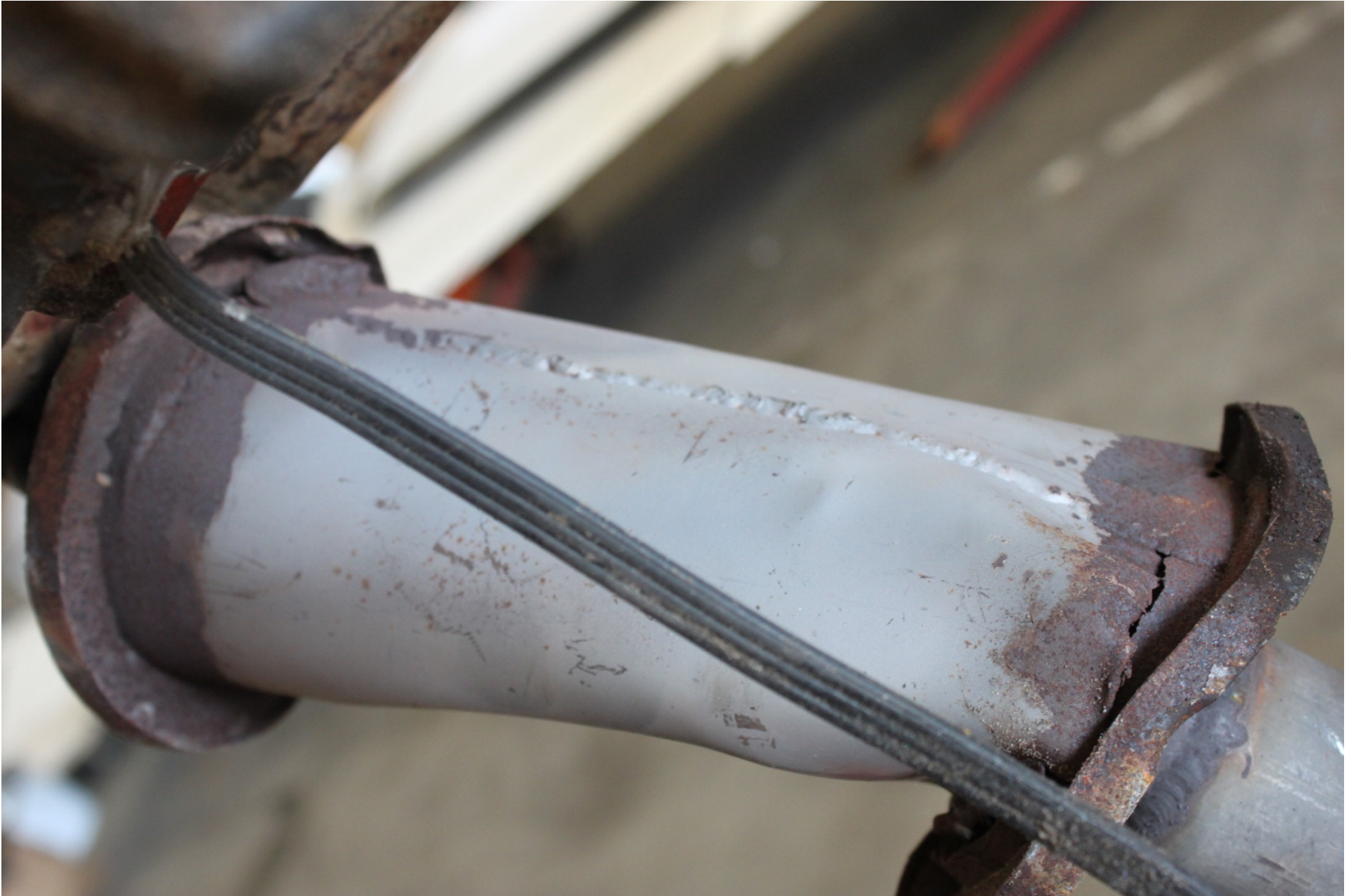
Photo 3 – Engine exhaust muffler, view #2
