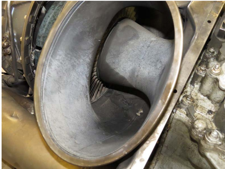
Interior of Exhaust Collector Support
