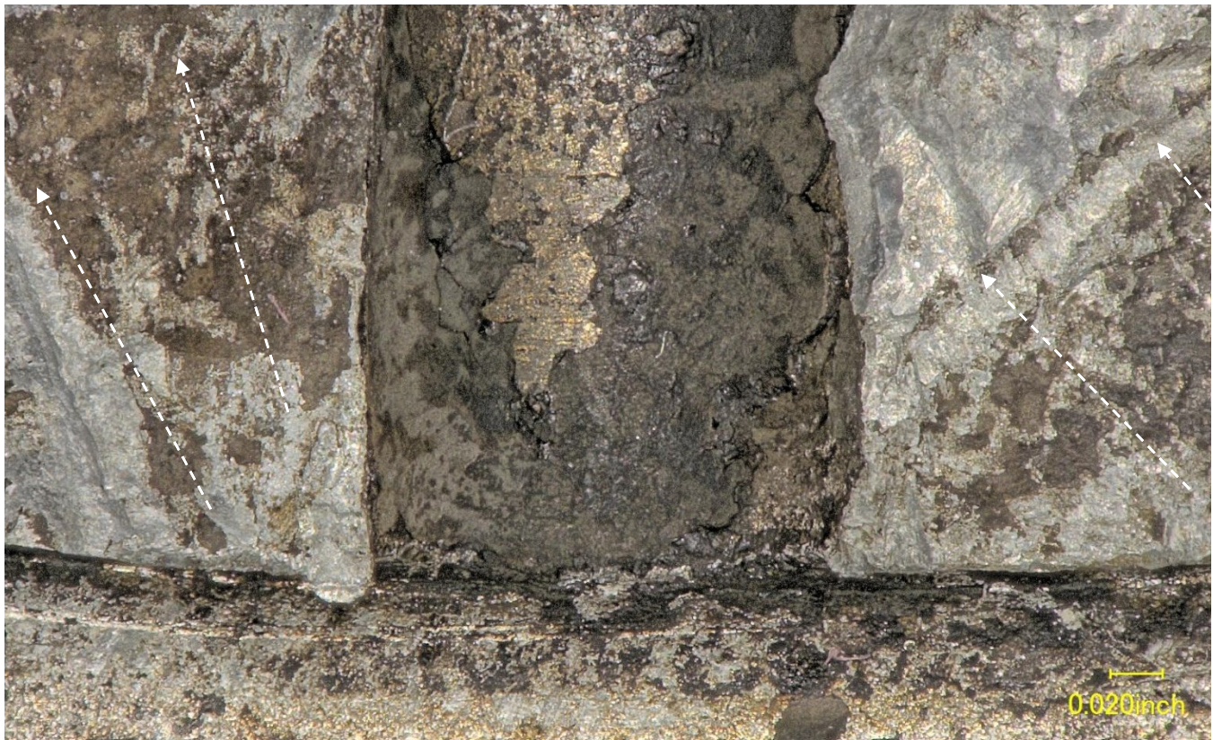
Figure 10 – Closer view of the oil hole in Figure 9, showing one of the crack initiations sites.
