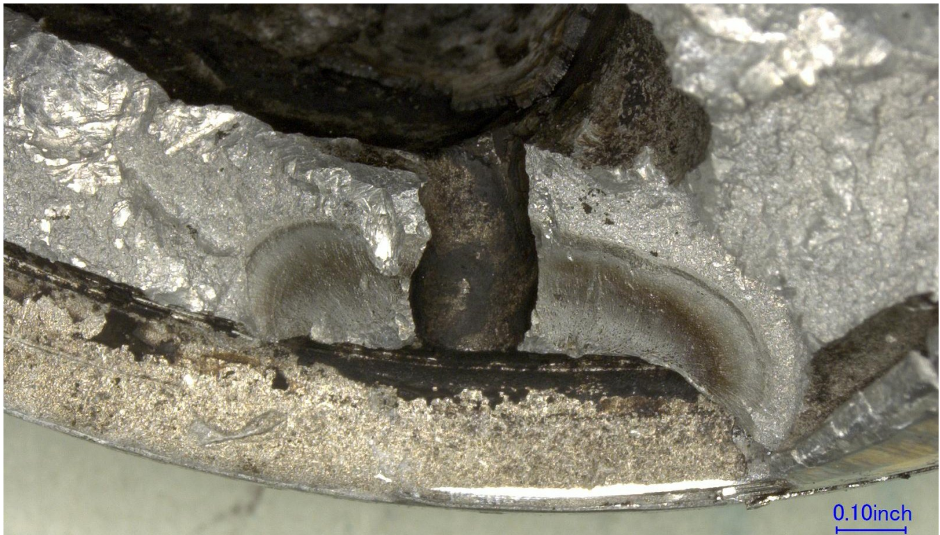
Figure 2 – Closer view of fatigue crack A, as labeled on Figure 1.
