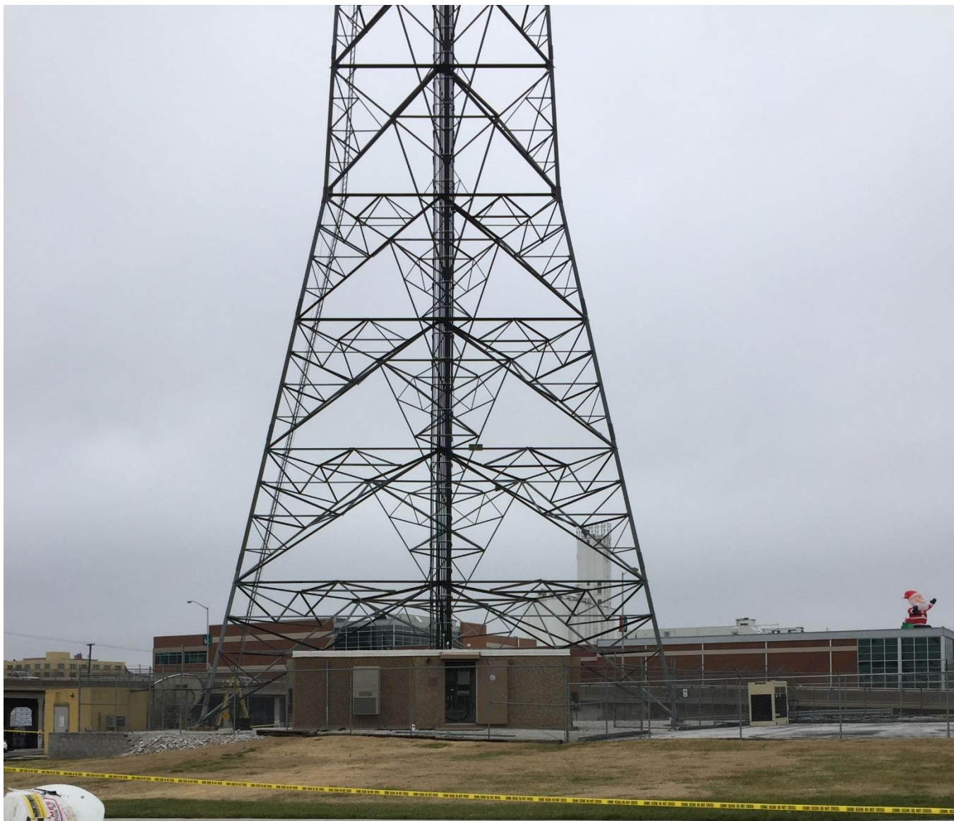
Photo 2 – Street level view of the base of cellular tower (FAA Photo)
