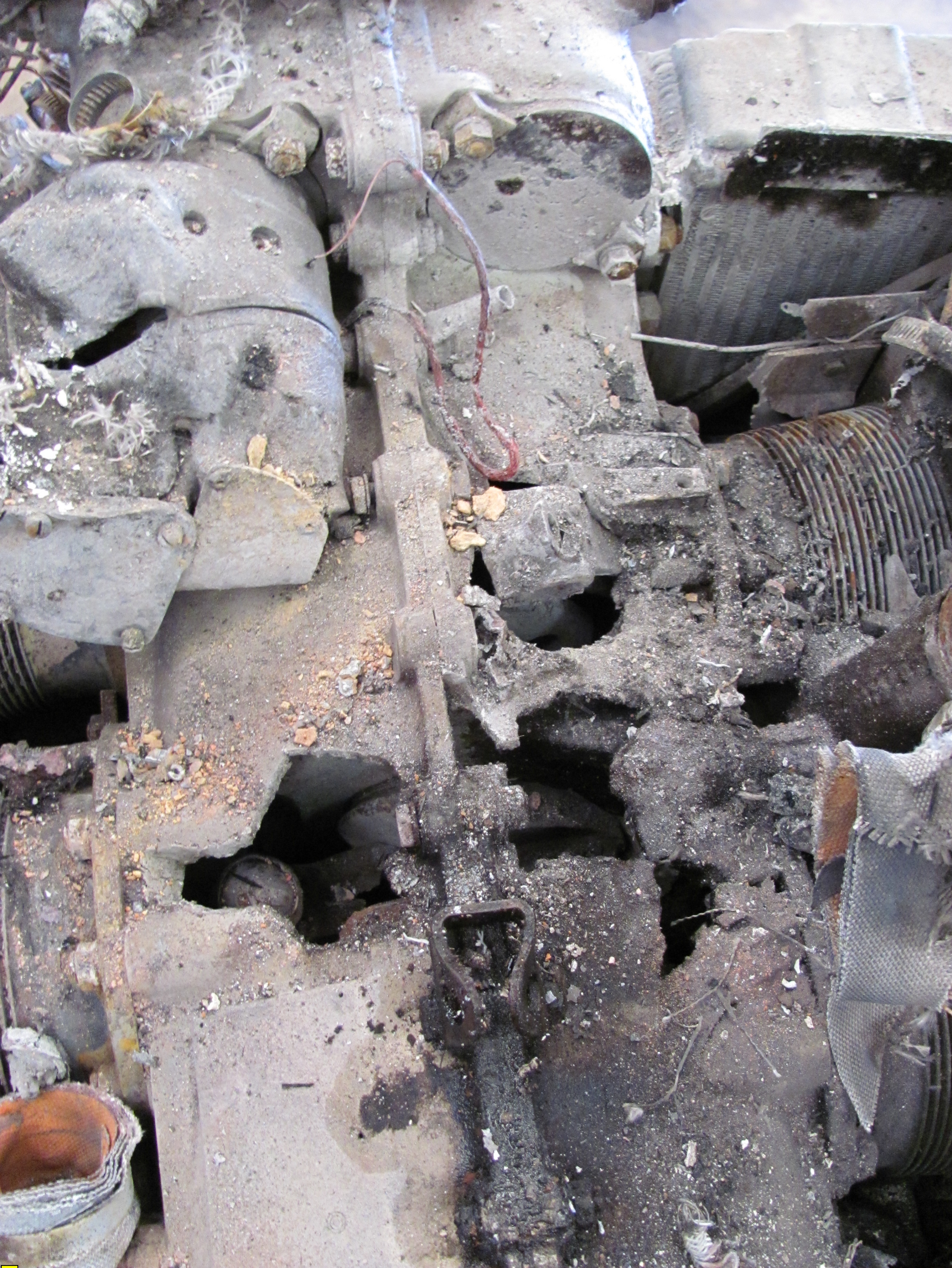
Photo 2 - Holes in Engine Crankcase (top view)
