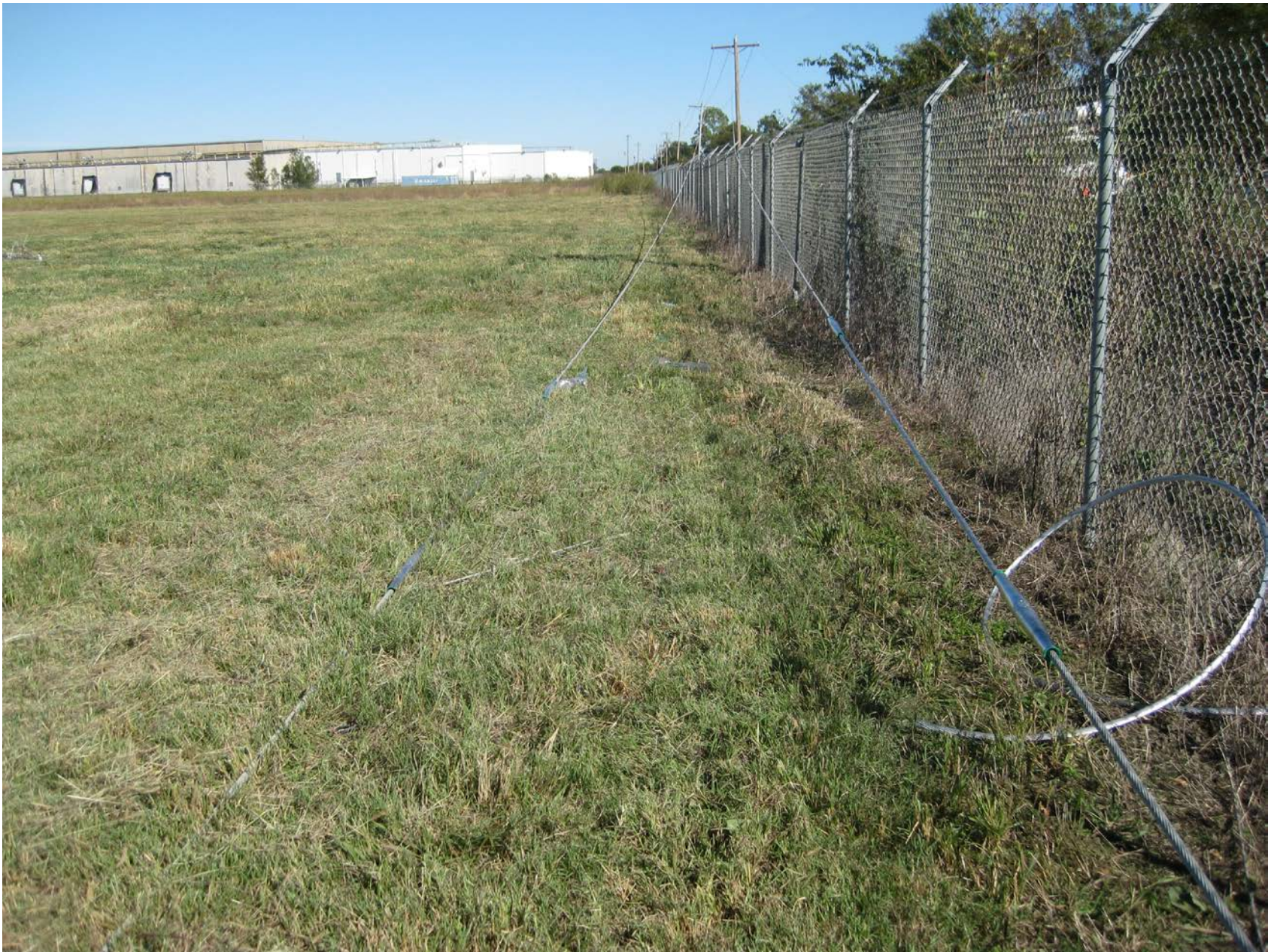
Photo 3 – Downed powerlines from airplane strike
