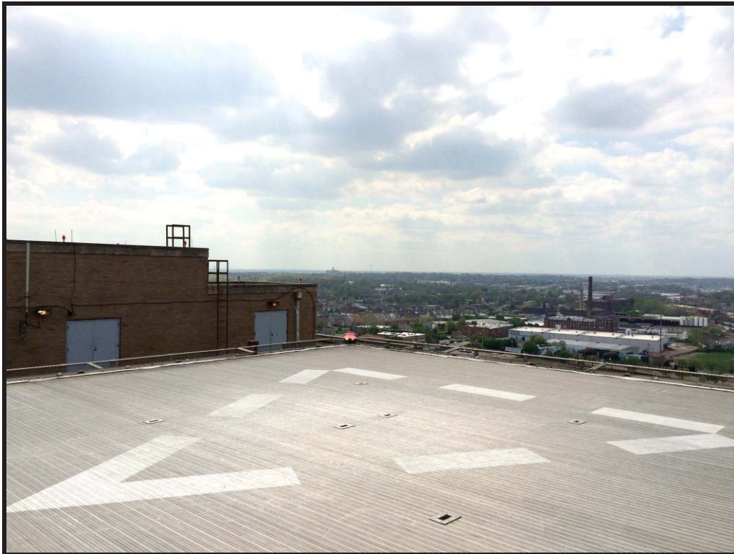
Figure 7: TLOF Overview, Looking SW
