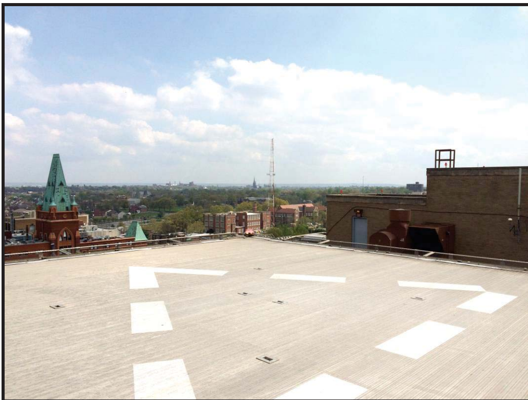
Figure 6: TLOF Overview, Looking SE
