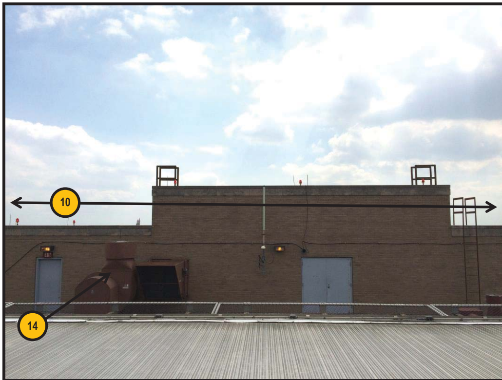
Figure 15: From TLOF Center, Looking S
