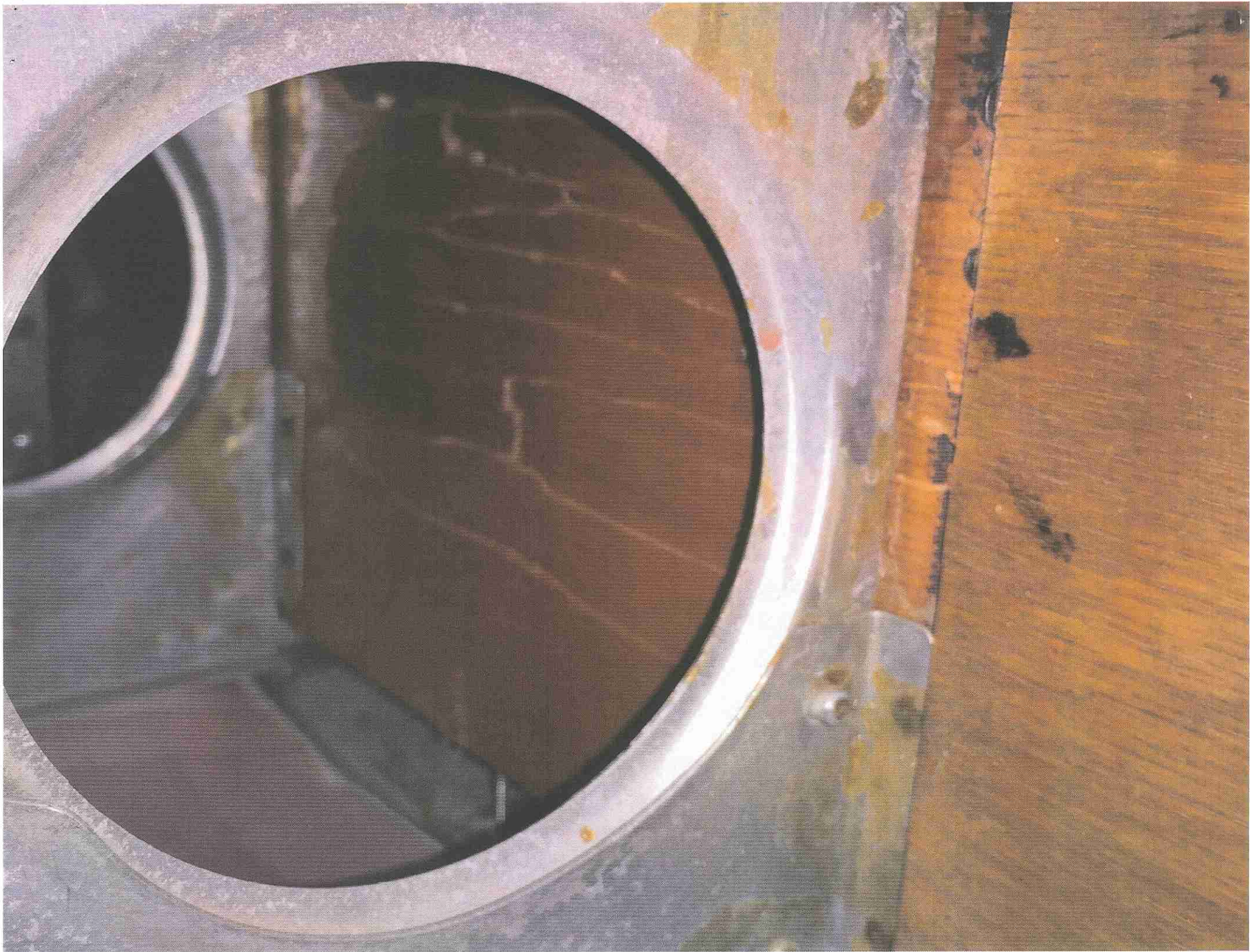
Photo 2 – Wing Spar Damage (Photo Courtesy of FAA)
