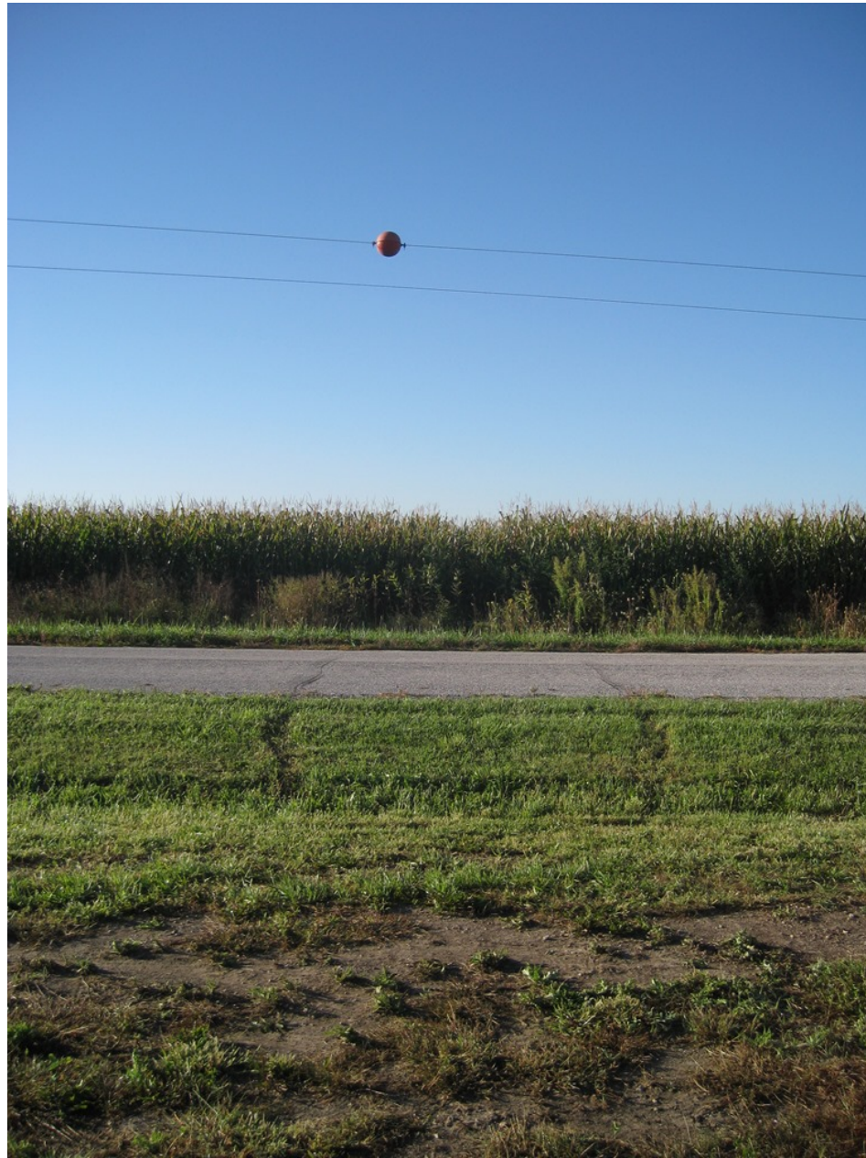
Photo 4 – Roadway Embankment and Powerlines
