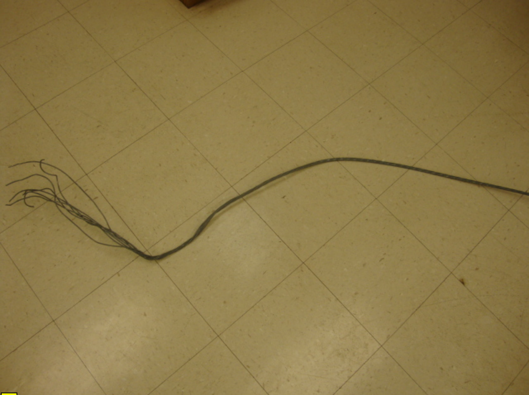
Photo 7 – Broken Static Line – West End (FAA Photo)
