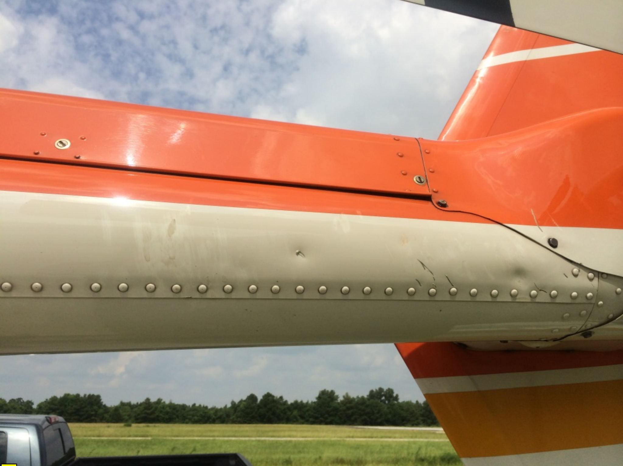
Photo 1 – View of tailboom damage
