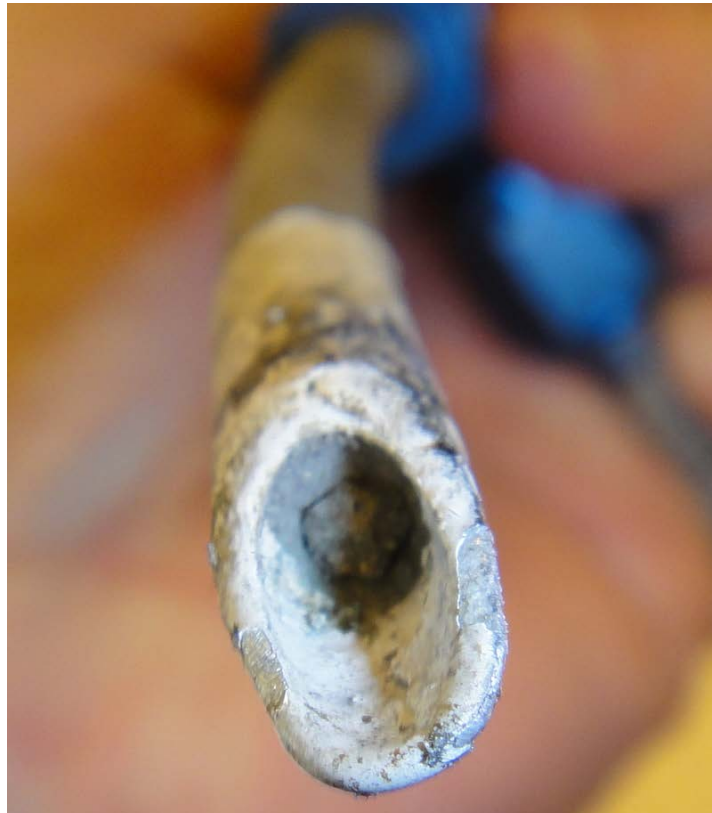
Figure 10. Close-up photograph of the end of the heater drain line.
