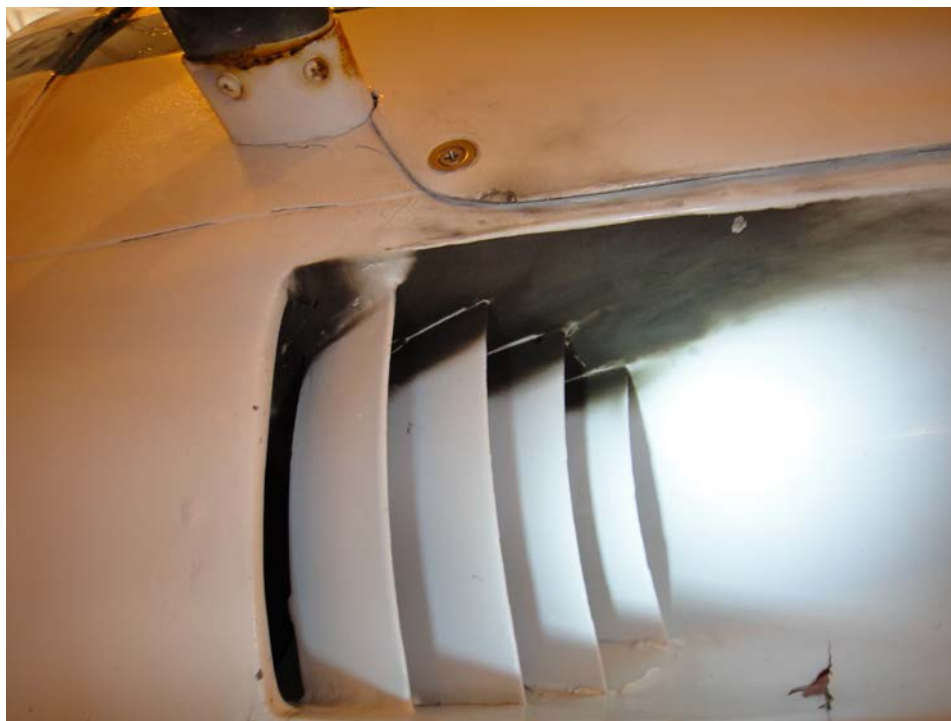
Figure 7. Close-up of sooting on lower right exhaust louver.
