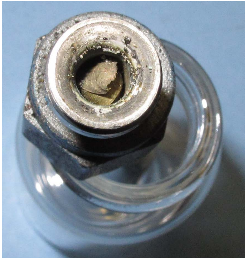
Figure 18. Close-up photograph of fitting end of cabin heater drain line (opposite end of line in Photograph 10).
