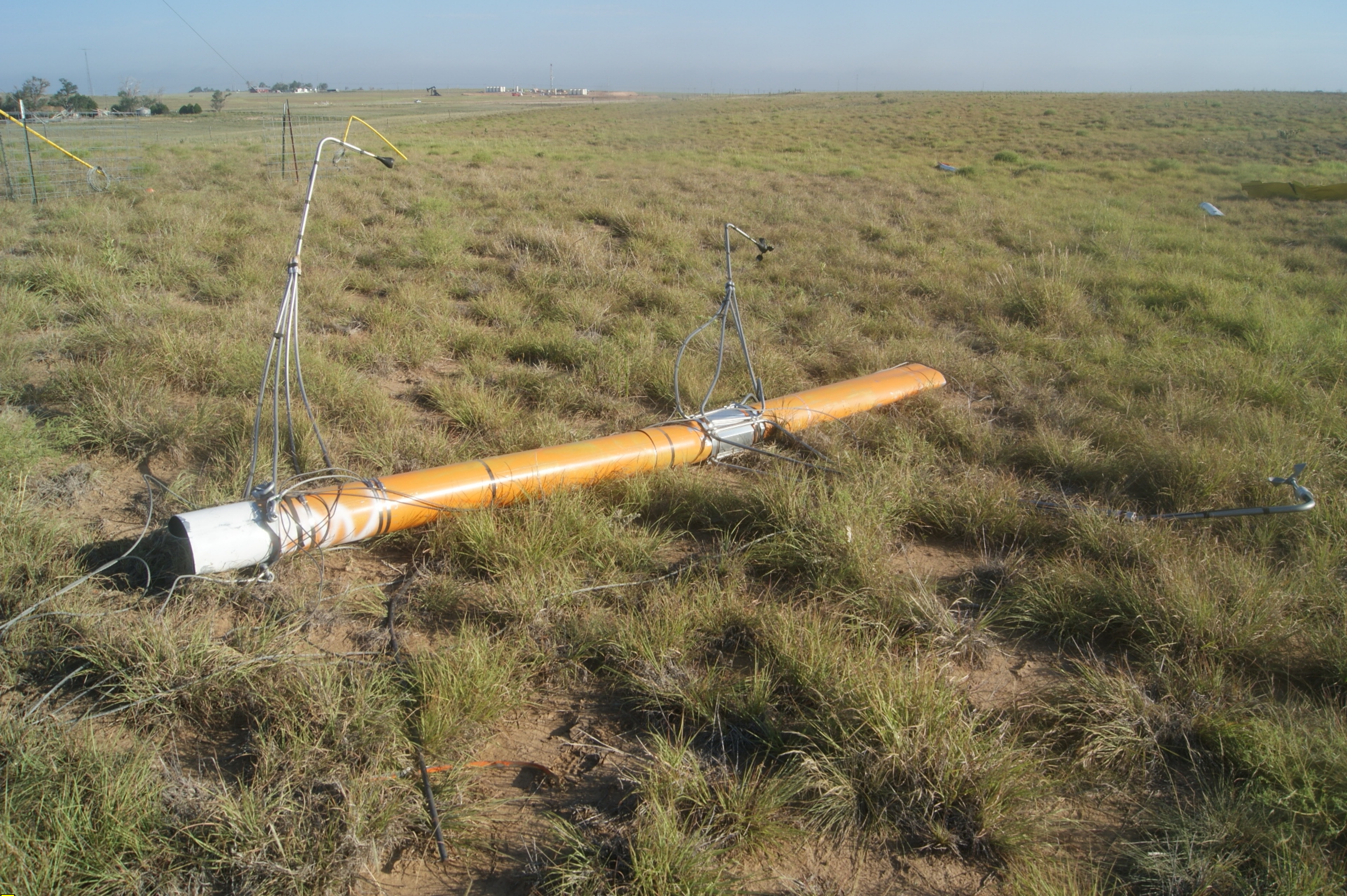
Photo 2 - Portion of severed meteorological tower.
