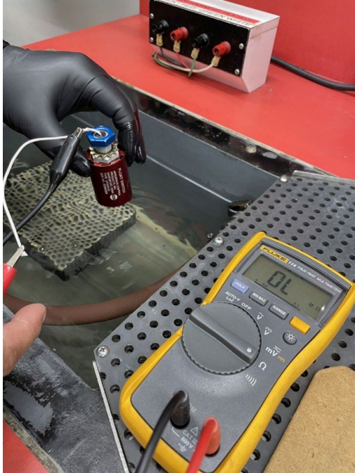
Figure 18 - Float switch in open position during testing (NTSB photo)
