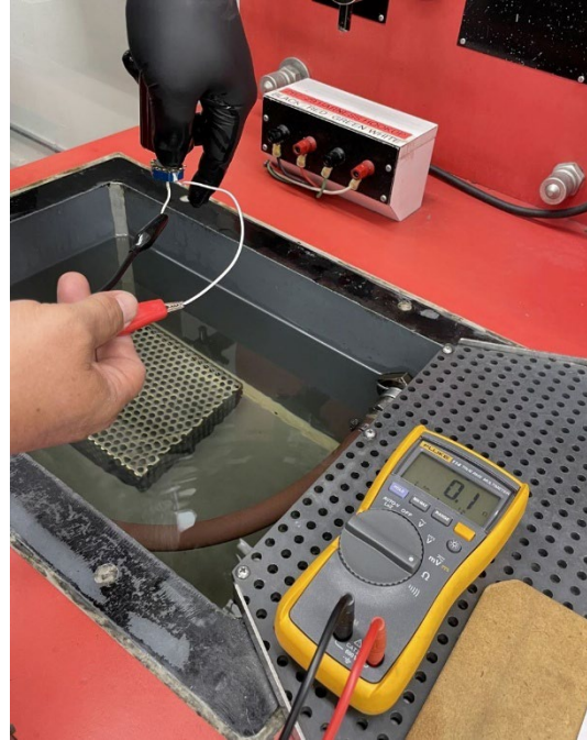
Figure 19 - Float switch in closed position during testing (NTSB photo)
