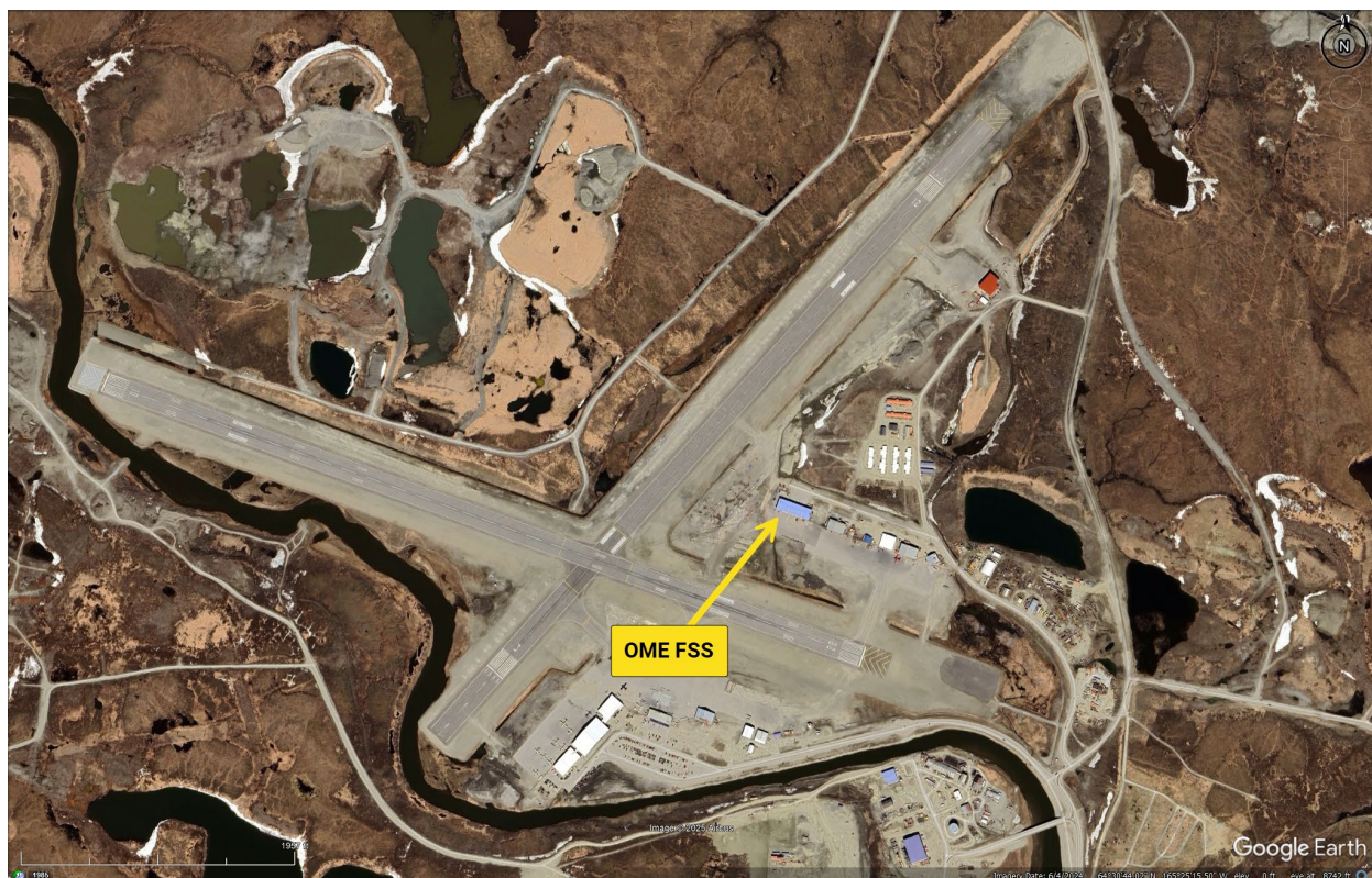
Figure 10. Google Earth Screenshot of OME FSS building at PAOM.
