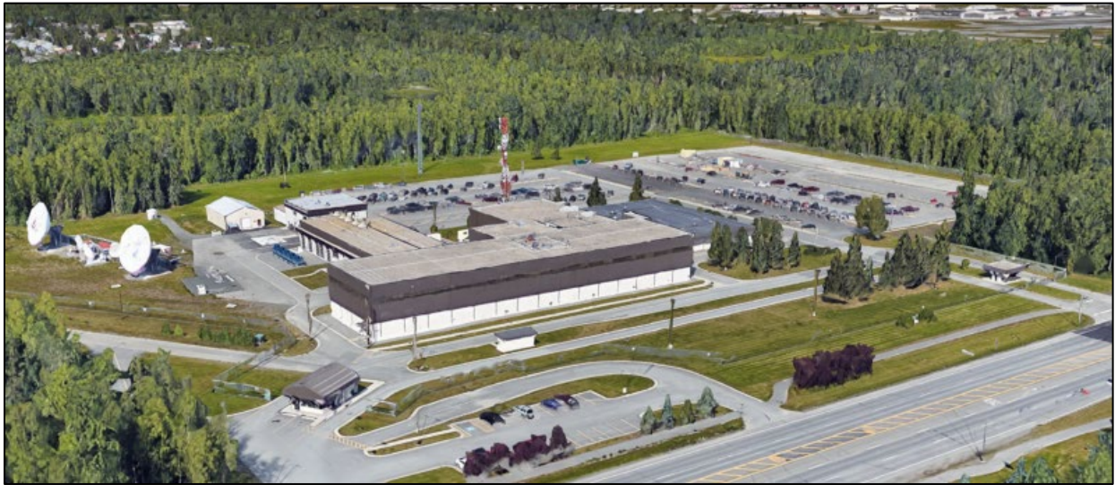
Figure 7. ZAN facility building. Photo credit: FAA.
