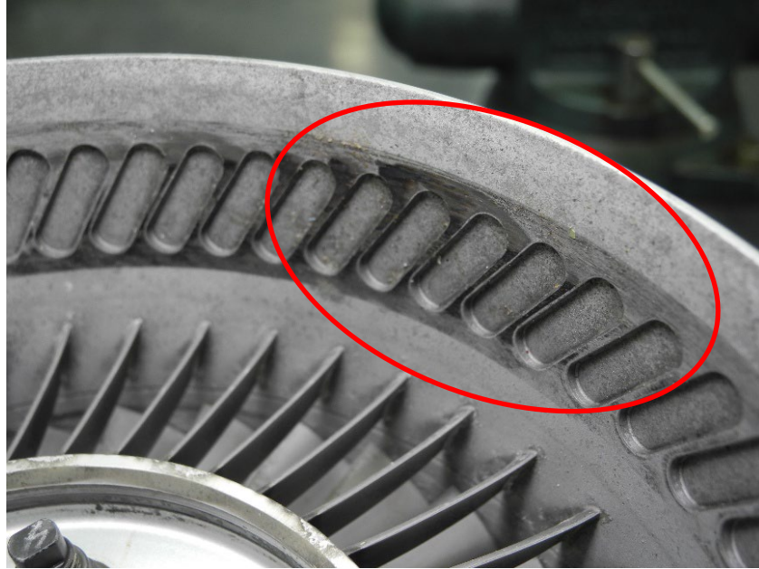
Photo 35 - 1 st Stage Compressor Shroud - Scored at 3 - 6 O'clock Position
