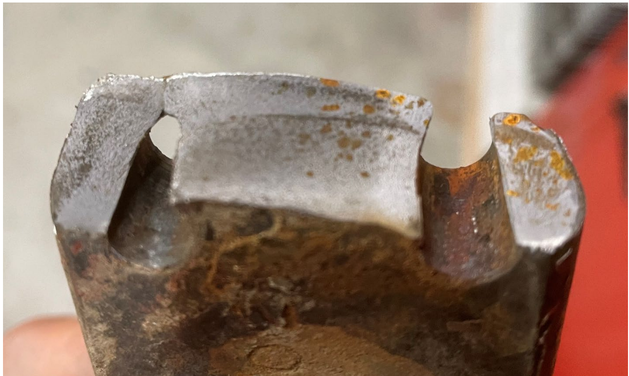
Figure 2. Corrosion on the inboard surface and in the forward hole (Photo by owner).
