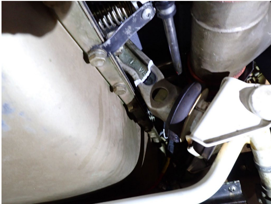
Figure 2 Broken engine mount
