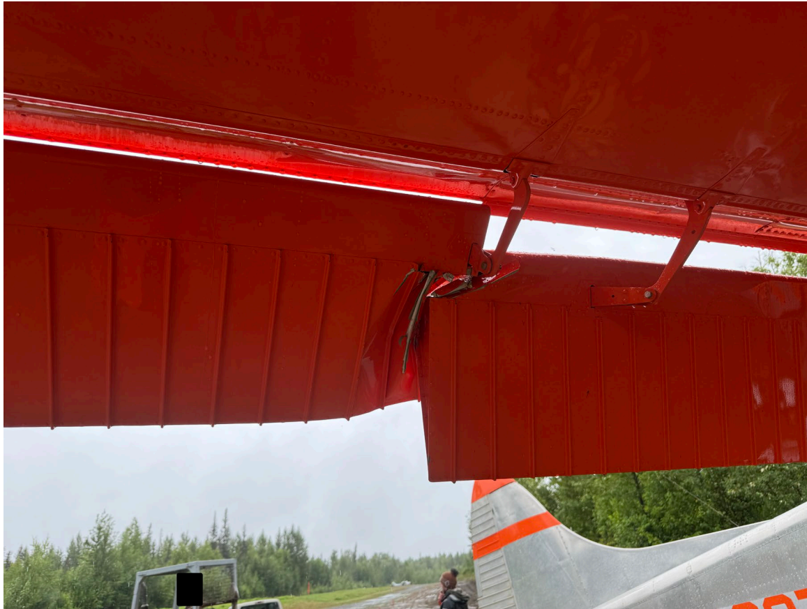
Photograph 3 - View of the underside of the right wing (Courtesy of owner)
