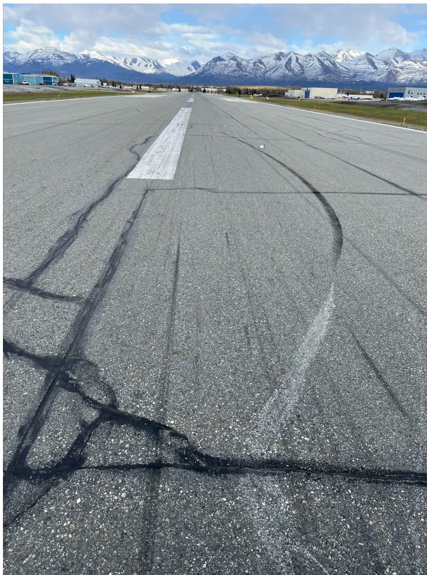
Photograph 4 - Marks from airplane propeller on runway (Courtesy of PAMR)
