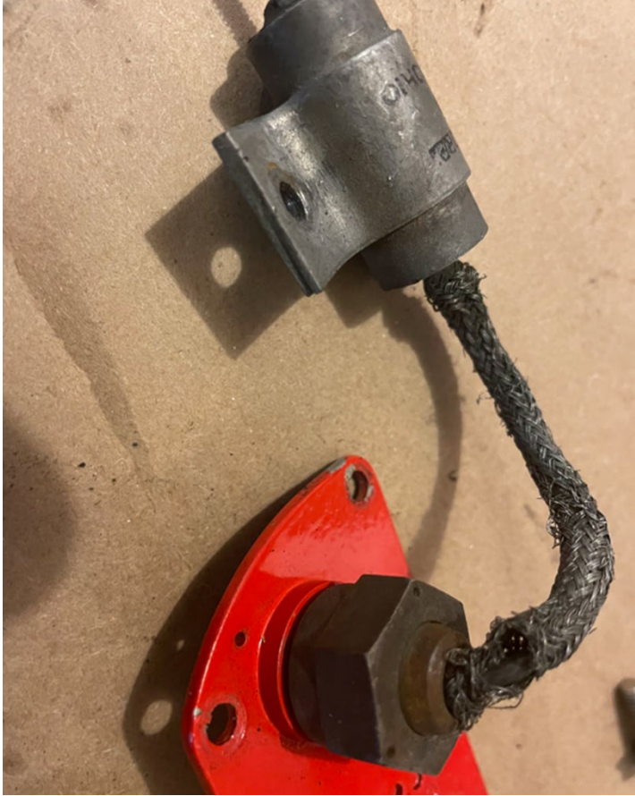
Figure 19 view of wire damage to the P-lead connection into the back of the left magneto.
