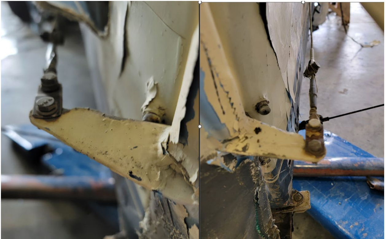
Figure 7 View of the flight control cables attachment to the rudder horn.
