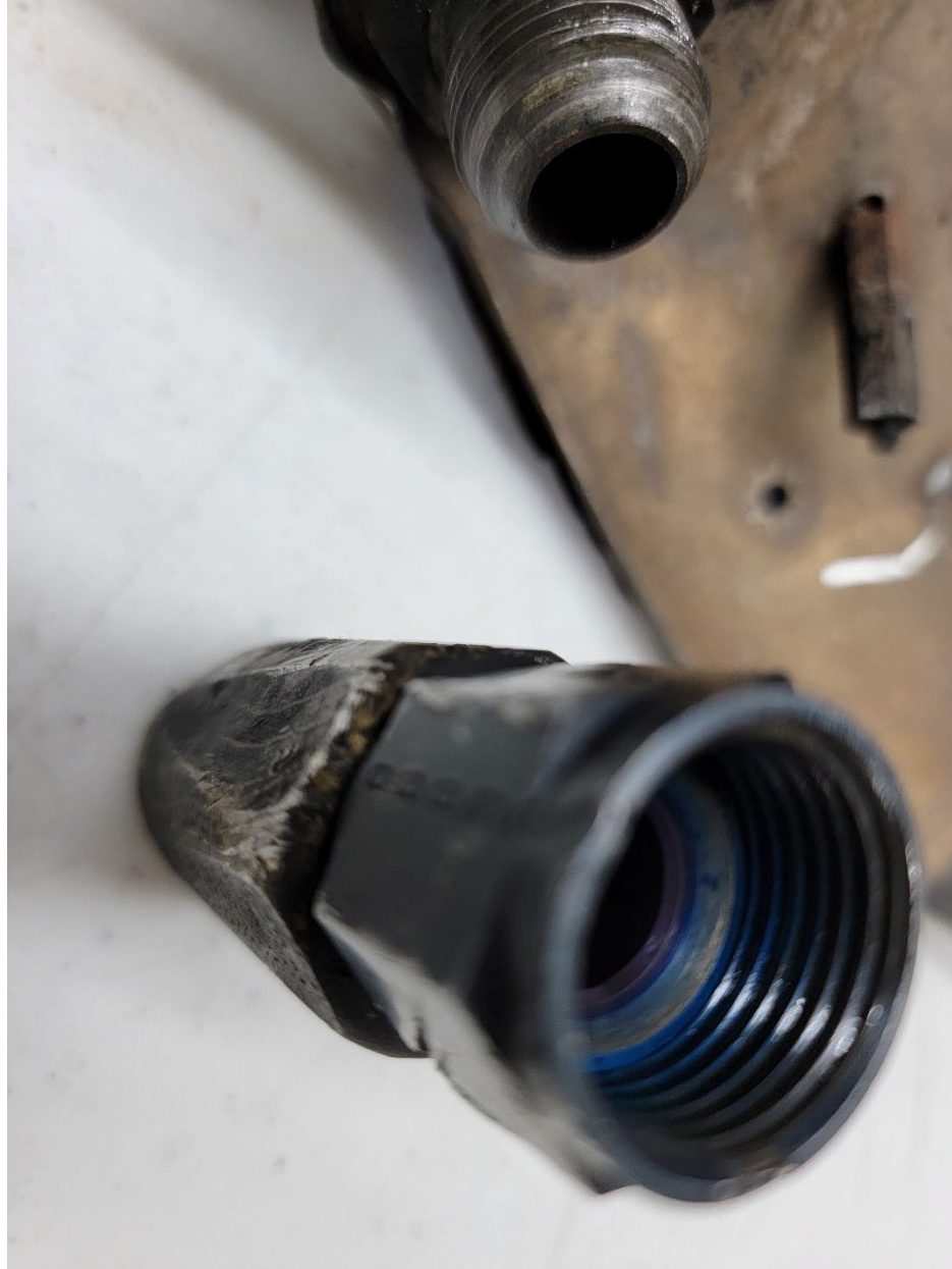
Figure 1 AN-8 hose fitting found in the exhaust heat shield with undamaged threads.
