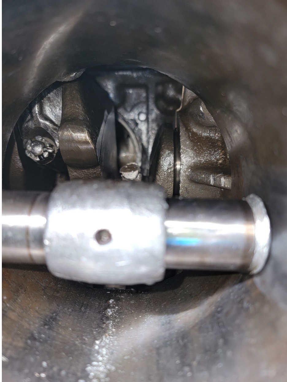
Figure 3 View into the engine case from the No. 1 cylinder.
