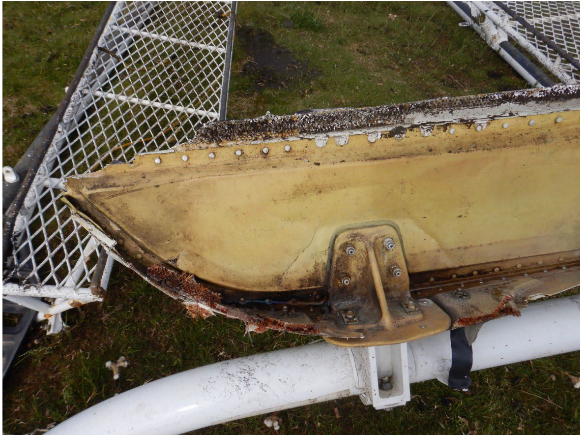
Figure 38 Rear view of the landing gear left attachment point.
