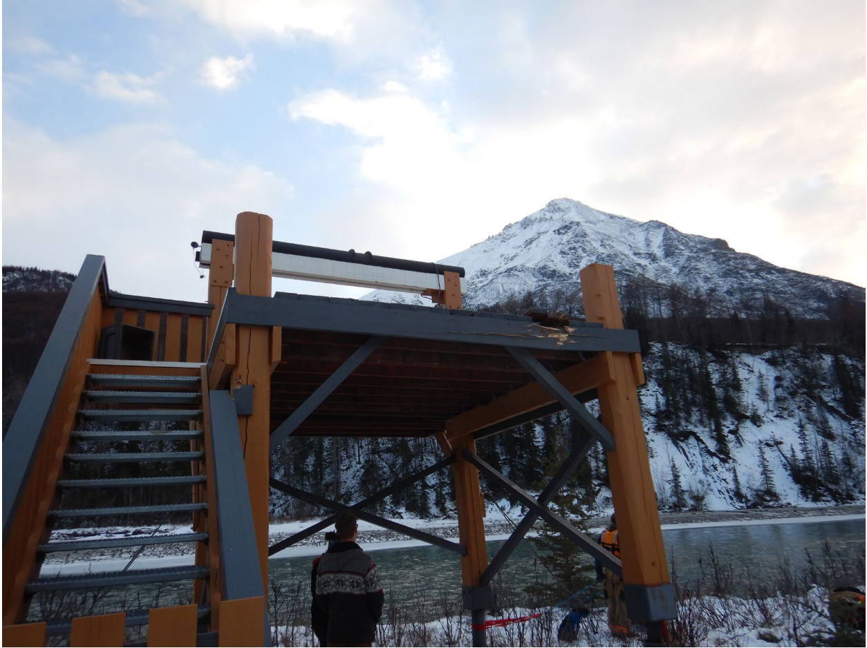
Figure 2 Cable attachment point on the north side of the river.
