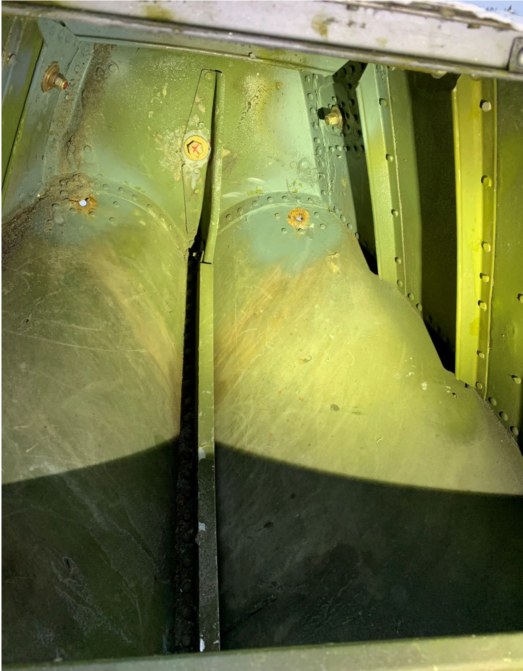
Figure 4 Inside the float locker. You can see the upper side holes were plugged but the lower center holes were open.
