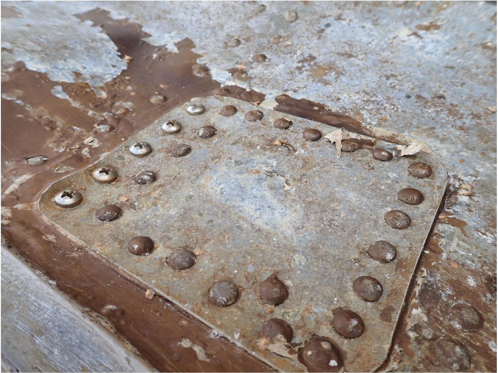
Photo 5 – View of patch and screws on the hull of the right float. (Photo courtesy of Textron)
