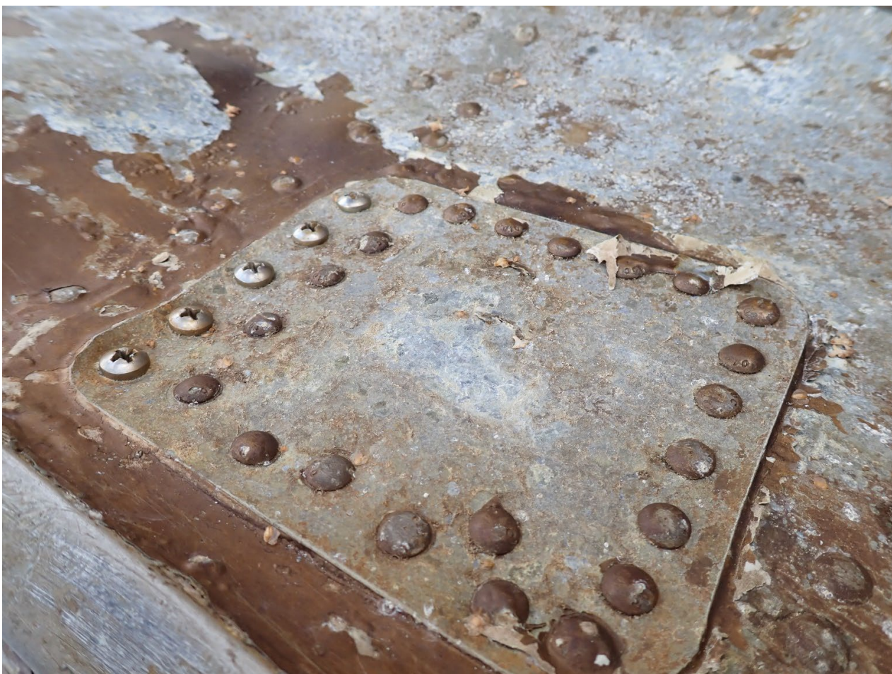
Repair to the hull of the right float, ASI-22-CI-072
